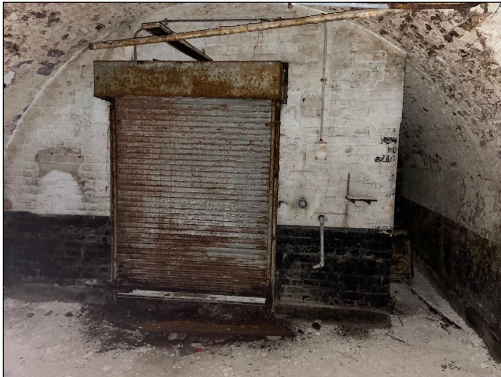
Figure 19: Example of a later enclosure to be demolished within the listed vaults
