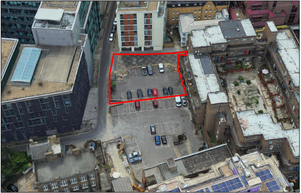
Figure 2: Aerial view of site (in red) from the north looking south
