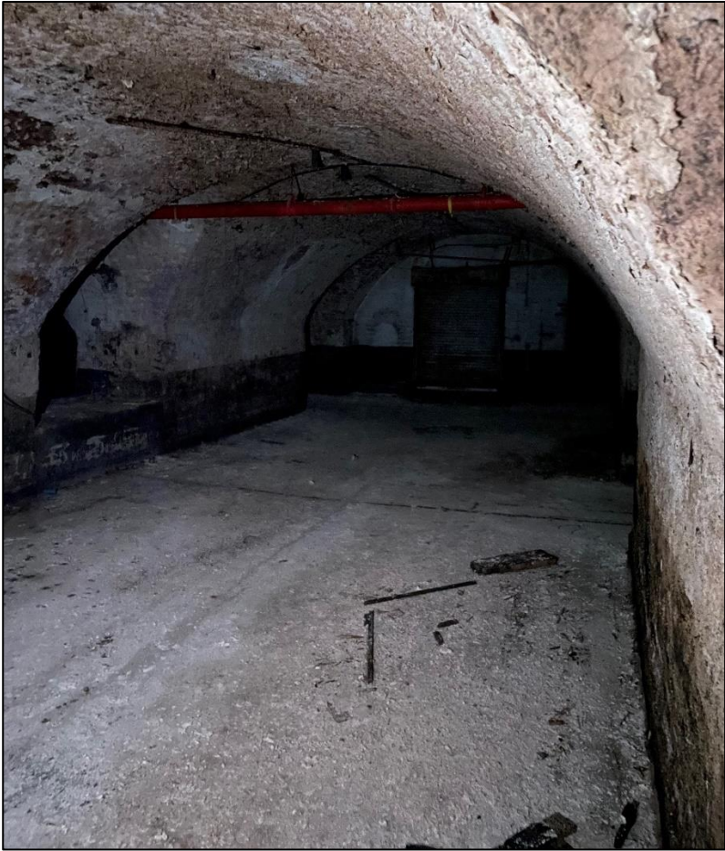
Figure 7: View of within the listed arched vaults at basement level
